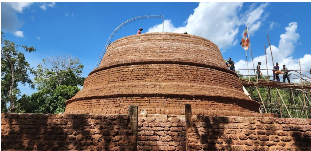
The stūpa conservation in progress
